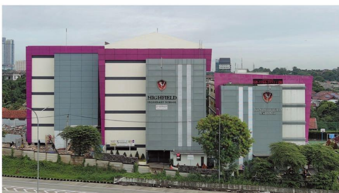
Highfield Secondary School - Depok
